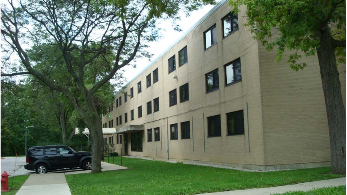
Figure 3 - Bldg 128H looking south
