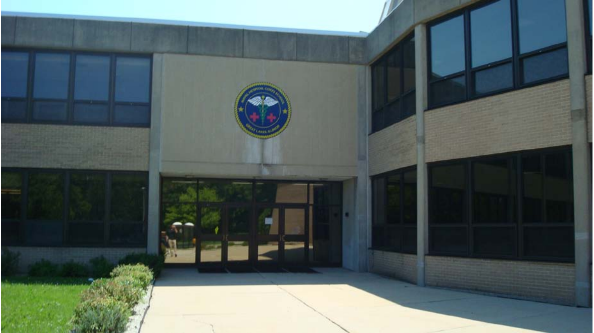
Figure 1 - Bldg 130H looking south
